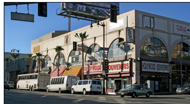
Before: Petersen Building prior to renovation
